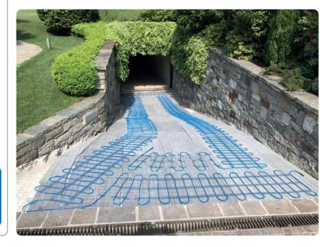
**ATTENTION:** since it is a constant power cable, the *EASY RAMP* can not be cut, jointed or overlapped.
