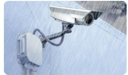
Installation with free cables.
