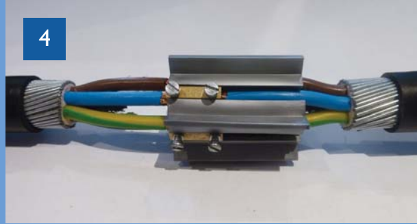
4 Insert the prepared cores into the connectors
